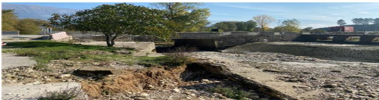
Figure 1: Images of Viroi Bridge
